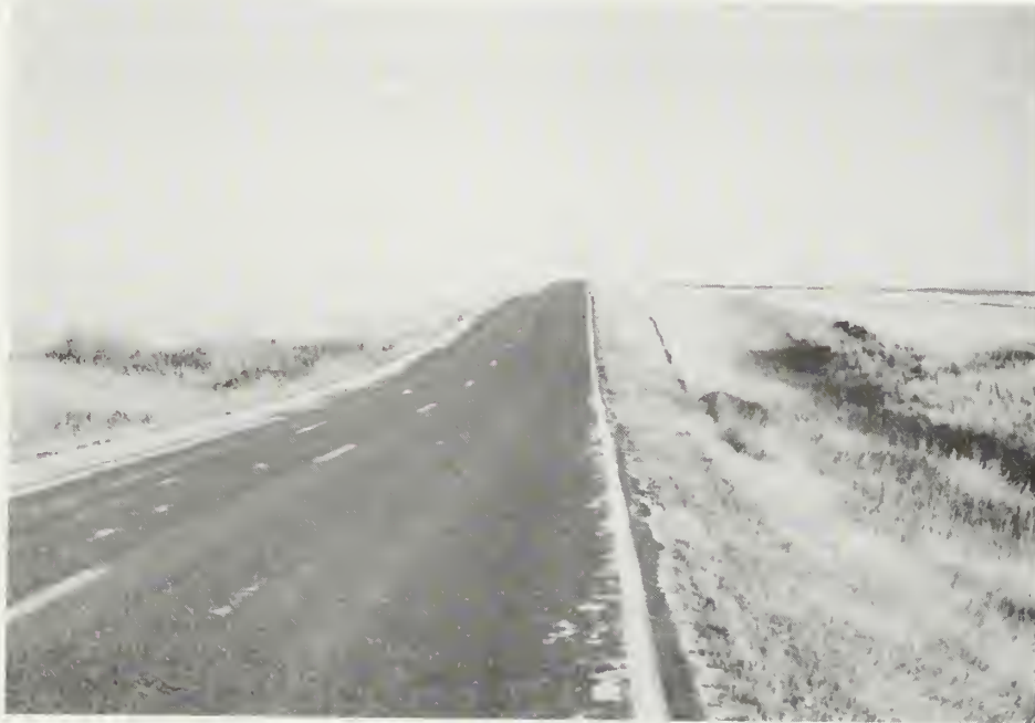
Figure 2 - North view near milepost 1
